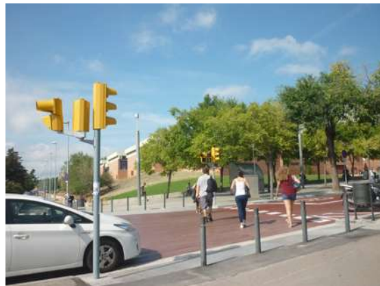
Fig. 2. Improved accessibility with new ramps on pedestrian crossings and the re-painting of horizontal signalling
