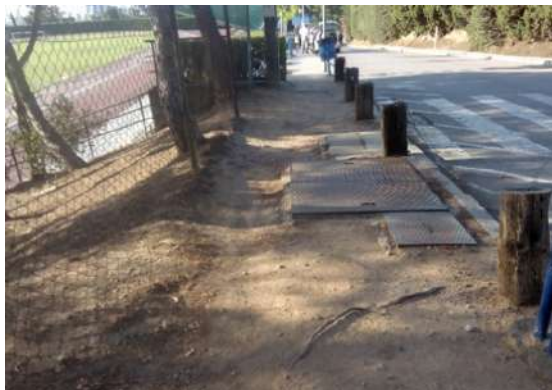
Fig. 5. Unpaved pathways in bad condition
