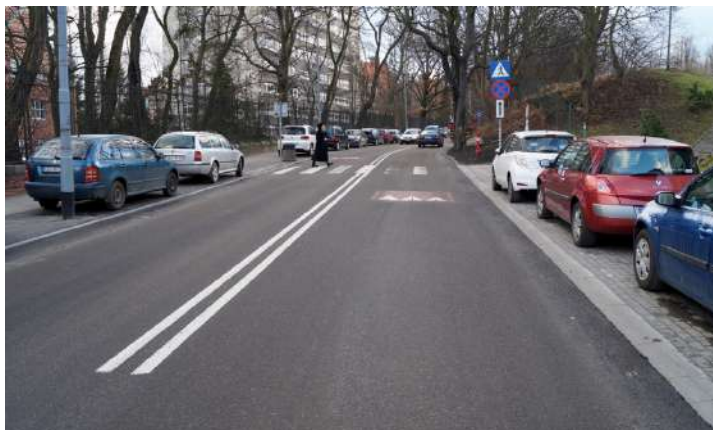
Fig. 2. Traugutta Street (from the Church of St. Nicholas to the crossroad with Sobieskiego Street) before renovation
