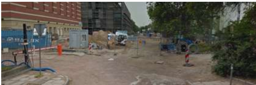
Fig. 1. Square in front of the Nanotechnology B Center - during renovation
