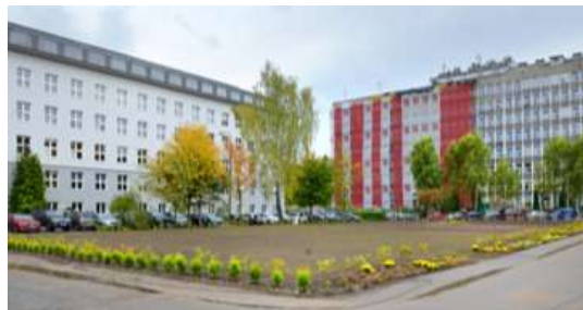
Fig. 2. Area after the investment - a combination of a green recreational area with a ground car park
