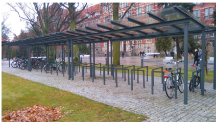
Fig. 3. A covered bicycle parking lot for bicycles in front of the main, historic building of GUT. Fot.: K.Janiszevska
